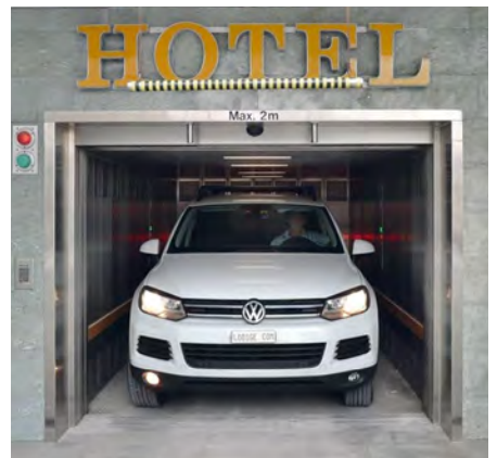
Garage Swissotel - Zurich, Switzerland
