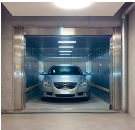
Underground car park - Zurich, Switzerland
